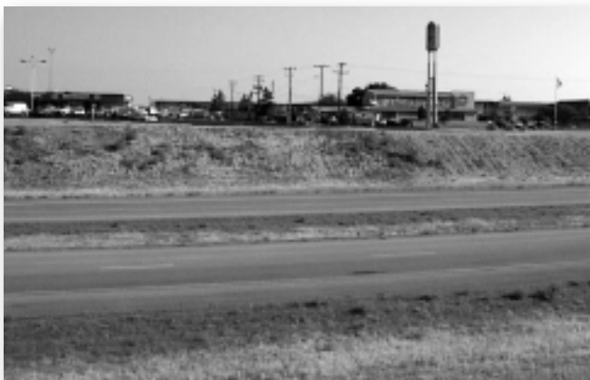
Figure 3 – Vegetation Established on Slope
