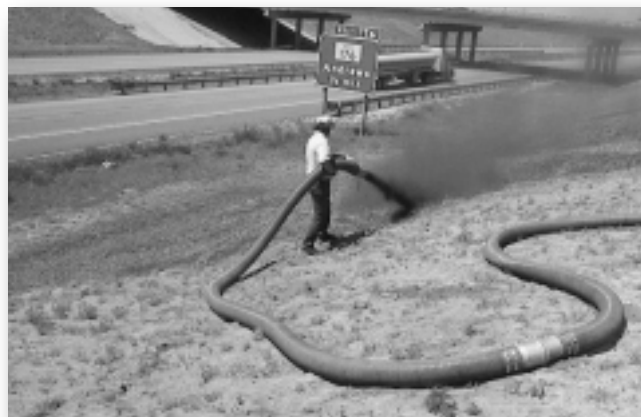
Figure 2 – Applying Compost
