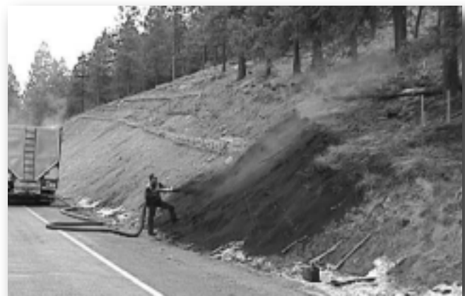
Figure 1 – Applying Compost (Chelan Site)
