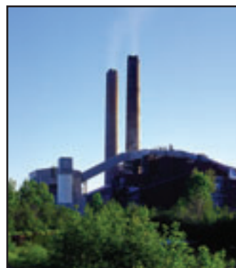
Marquette Power Plant
