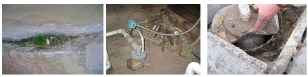
Cracks on a storage tank Rat droppings around the wellhead Seal on wellhead not watertight Photos courtesy of Nevada Division of Environmental Protection
