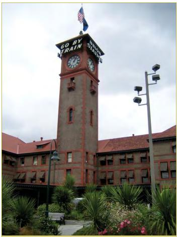
**Union Station** is an active Amtrak and freight station. TE-funded repairs were completed on the roof, masonry, doors, and interiors.
