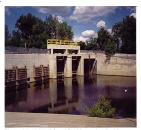
Figure 3.1: Hubbell-Southfield Retention Facility Overflow Gates
