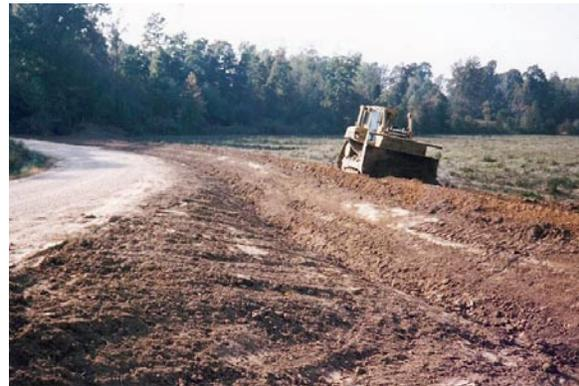
Figure 1. Re-grading channel banks and installing a levee along a rapidly eroding drainage area prevents agricultural field runoff from entering Dry Creek.
