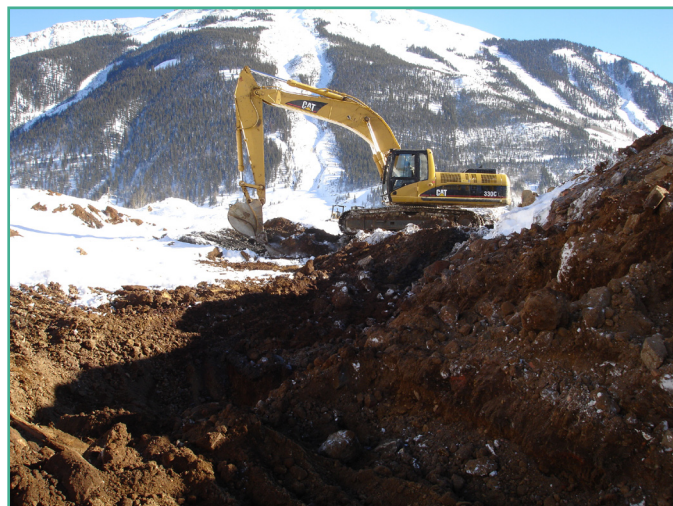
Cleanup underway at the Martha Rose/Walsh Smelter site.
