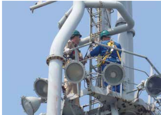
Measurement study at Indonesia's Star Energy KRA Platform
