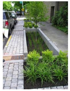
Figure 8. Another of the City's stormwater planter systems, installed next to a parking lane, includes a path of pervious block pavers for pedestrian access.
