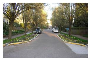
Figure 4. The landscaped curb extensions on Siskiyou Street improve aesthetics, calm traffic, and capture and infiltrate runoff from the street.
