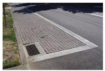
Figure 9. The curb lanes of Westmoreland Street were retrofitted with interlocking concrete block pavers. Excess stormwater not captured by the permeable pavement will overflow into existing stormdrain inlets, such as the one pictured here.
