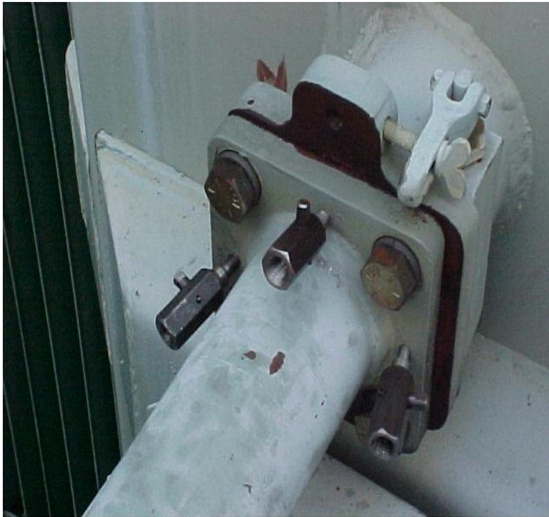
A Flapper Valve Flange That Has Been Drilled & Tapped - Ready For Injection
