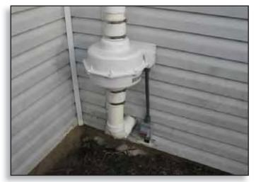
A vapor abatement system fan installed outside the house to remove contaminated vapor.
