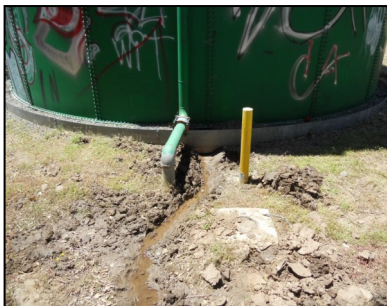
Before improvements were made, the tank had several leaks which can affect storage capacity and introduce bacteria into the system. Photo: Josh Newcom, IHS STARS database
