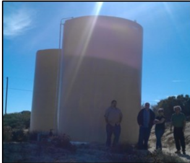
The project, which includes the two newly installed water tanks above, was completed in FY13. Photo: EPA
