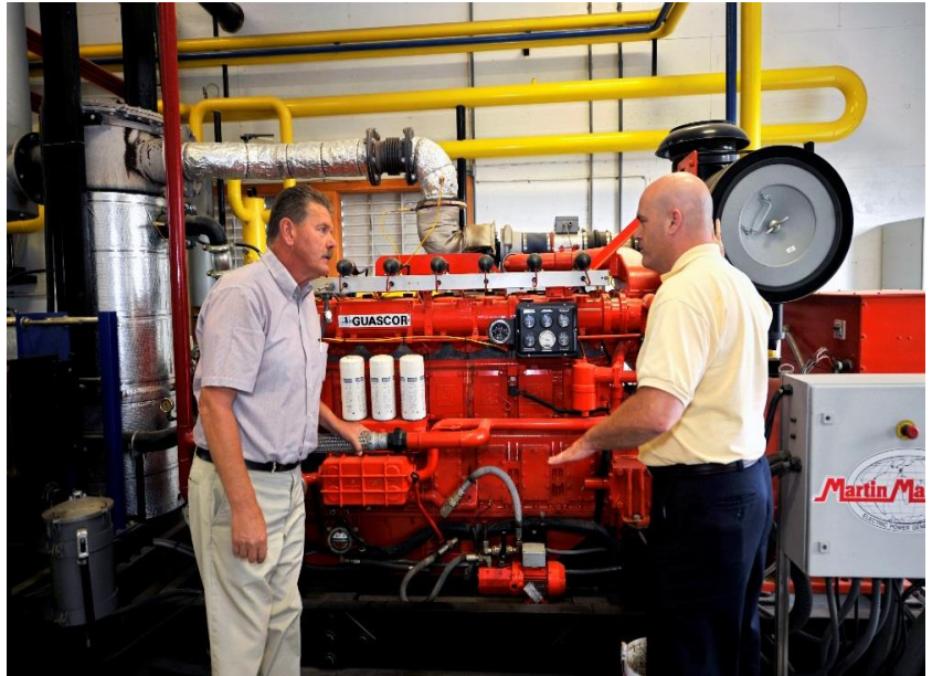
Photo: Bill Rowell of Green Mountain Dairy (left) and David Dunn of Green Mountain Power utility (right) discuss a biogas generator-set in Sheldon, VT.
