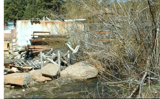
Before Placer County officials could restore the native wetlands at Snow Creek, debris piles from concrete production had to be cleared away.
