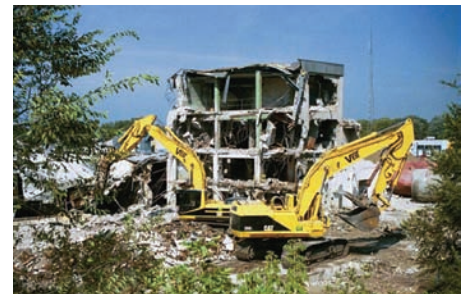
Conventional demolition underway.
