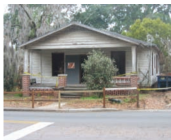
Wesley House prior to deconstruction (left). Deconstructed building materials from the Wesley House such as brick (center) and heartpine lumber from the main floor beams (right) used to build the library and lobby of the new Reichert House.
