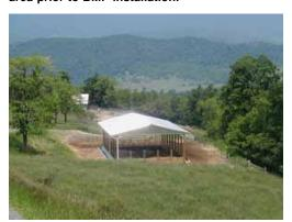
Animal feeding area after installation of waste storage facility, runoff control system, stream fencing, clean water diversion, paved feeding area, livestock watering facility, stabilized access road, and critical area planting.
