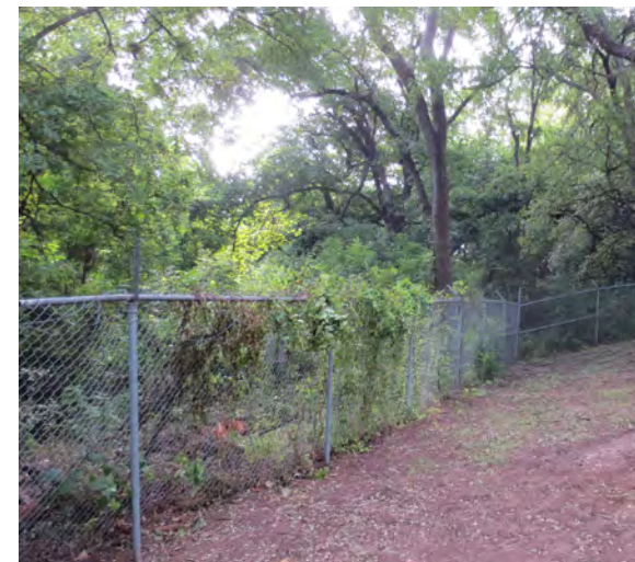
1 Figure 38 The Texas School for the Deaf campus's northern boundary. The fence also marks the top bank of Bouldin Creek.
