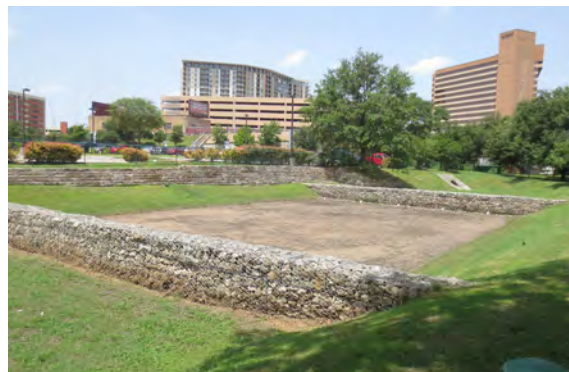
3 Figure 27 Typical stormwater infrastructure treating runoff from the Austin-American Statesman parking lots. The area is fenced with no public access.
