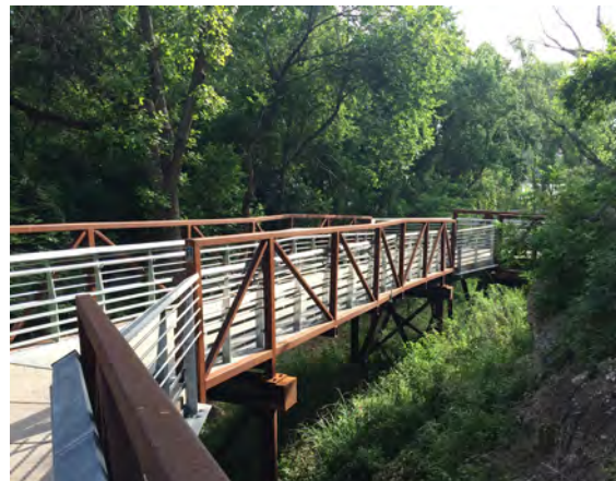
Figure 103 The Boardwalk at Lady Bird Lake could be a good model for the pedestrian and bike bridges spanning the creek.
