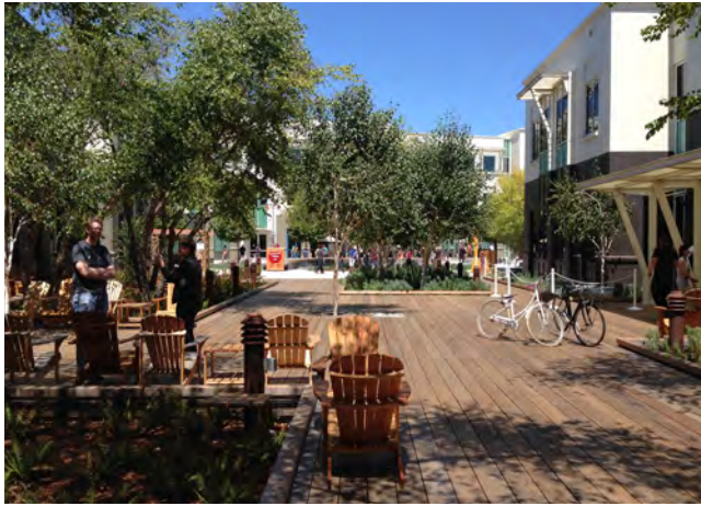
Figure 94 Pedestrian boardwalk over stormwater treatment gardens.
