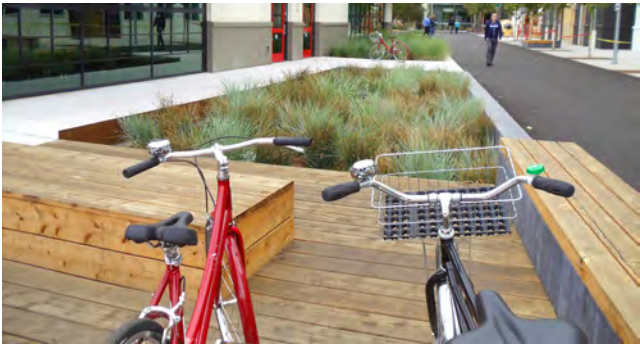
Figure 95 Pedestrian boardwalk over stormwater treatment gardens.
