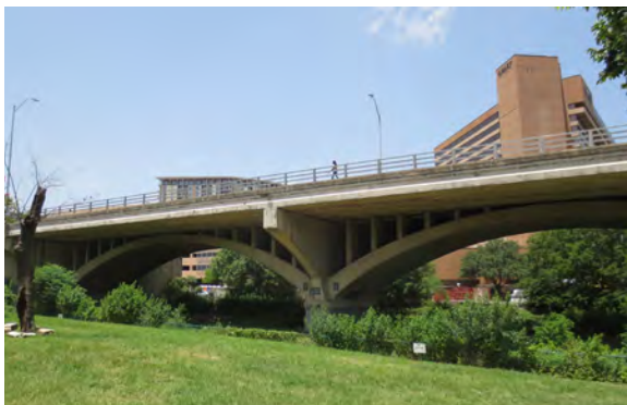
2 Figure 26 Austin-American Statesman property looking west toward the Congress Avenue Bridge
