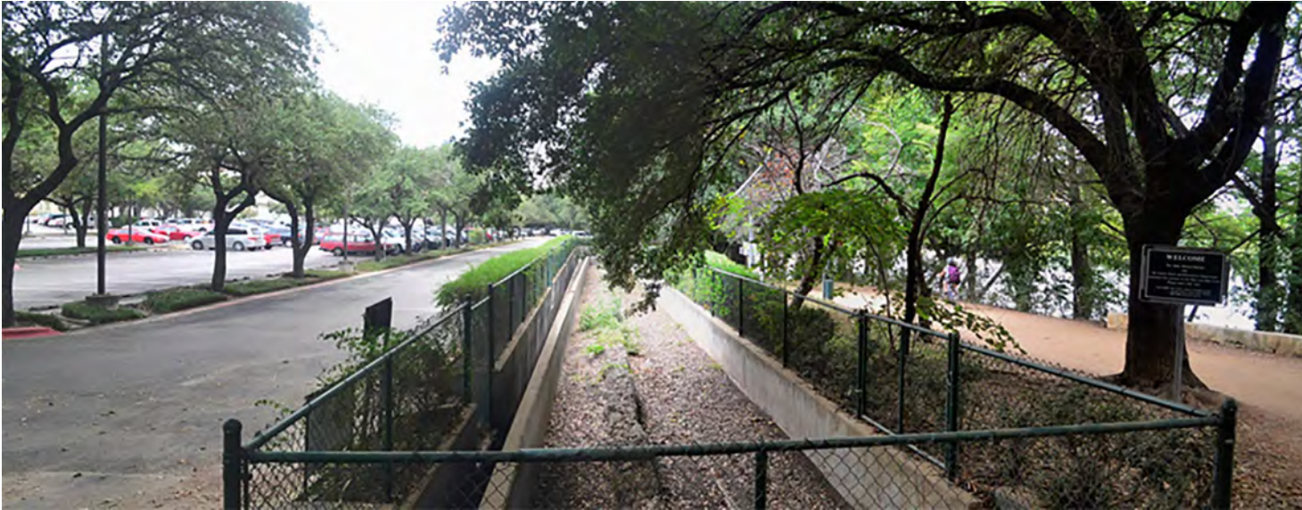
Figure 82 A sedimentation-filtration water quality pond occupies the site. Its built edges and fenced enclosure form a barrier to the park. A water quality pond that was more aesthetically and ecologically designed could be a park amenity rather than a barrier.
