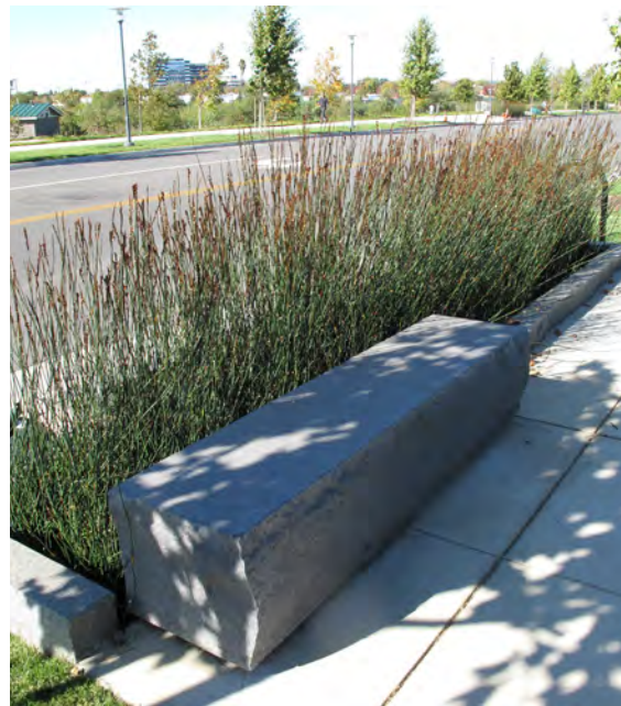
Figure 59 Flow-through planter for treating stormwater, with seating combines green infrastructure with streetscape furnishings
