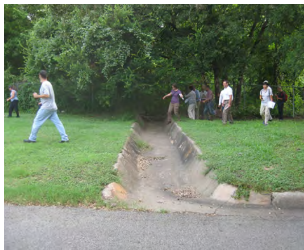
2 Figure 39 A concrete channel discharges stormwater runoff from the Texas School for the Deaf into the creek.
