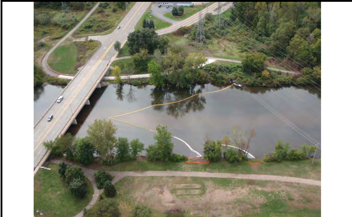
Photo Plate 3: Chevron Booming System
