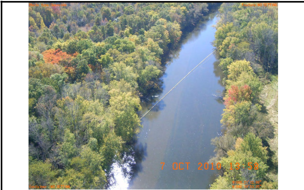
Photo Plate 1: Shore to Shore Booming System
