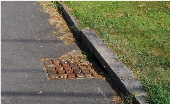
Photo credit: Tetra Tech, Inc. Figure 2-6. Slotted grate inlet catch basin
