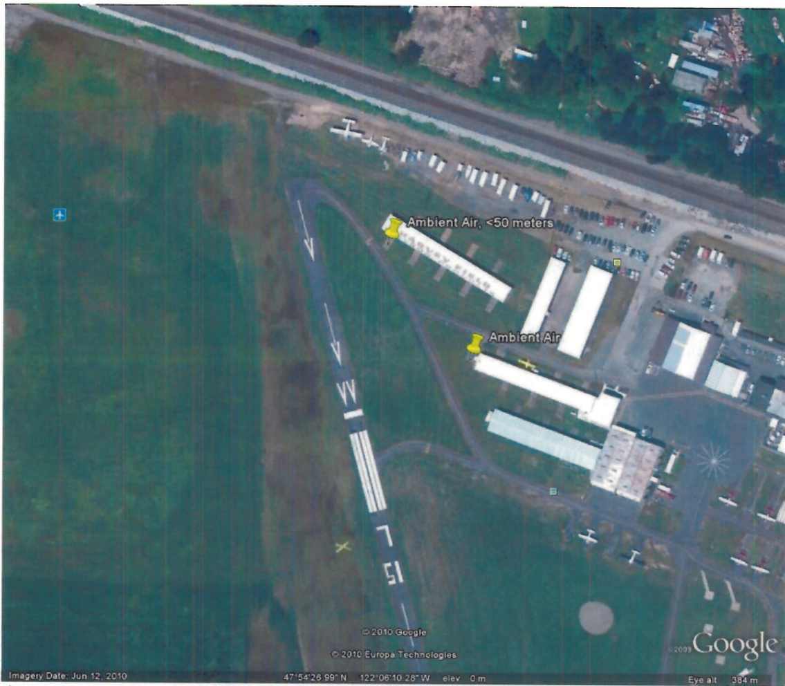
Figure 7: Ambient Air at Harvey Field near Runway 15
