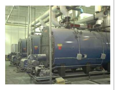
Seasonal, Oil-fired ≤ 5 MMBtu/hr, Limited-use, Boilers with oxygen trim systems that maintain optimum air-to-fuel ratio
