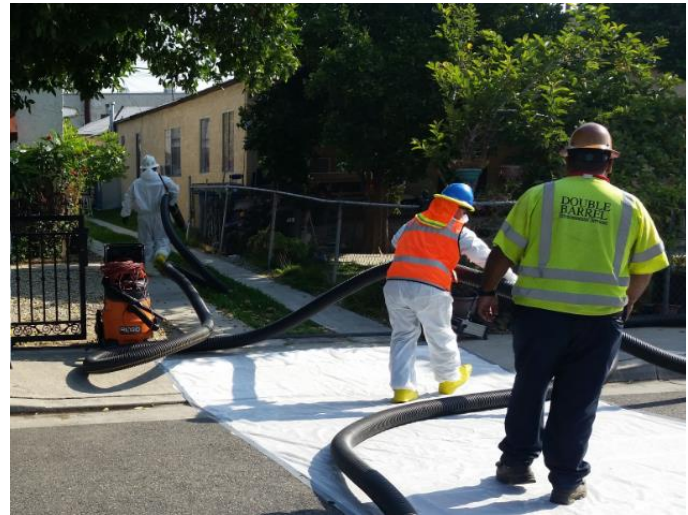
Figure 2: Cleanup crews removing ash from residential property exterior on E. 52 nd St.
