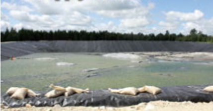
Lystek's 55,000 cubic metre lagoon holds 8,000 cubic metres of organic material
