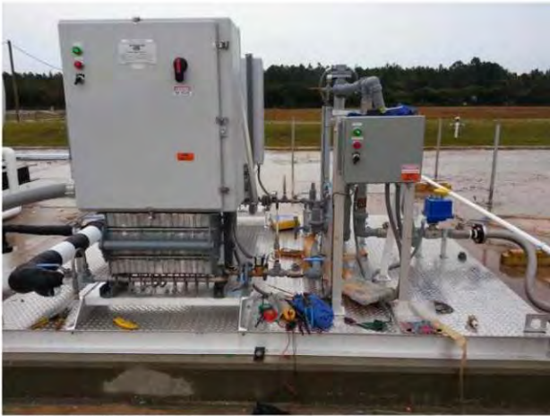
Left: 105-kW process vaporizers.
