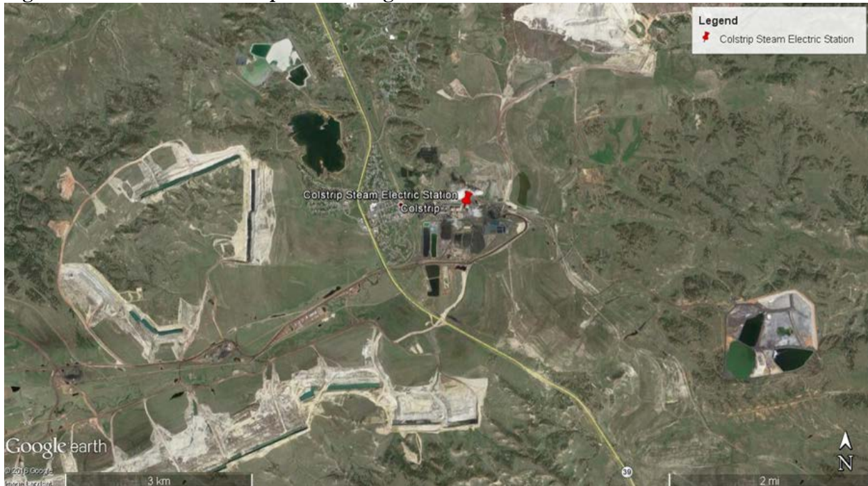
Figure 4. Aerial View of Colstrip Surrounding Area.
