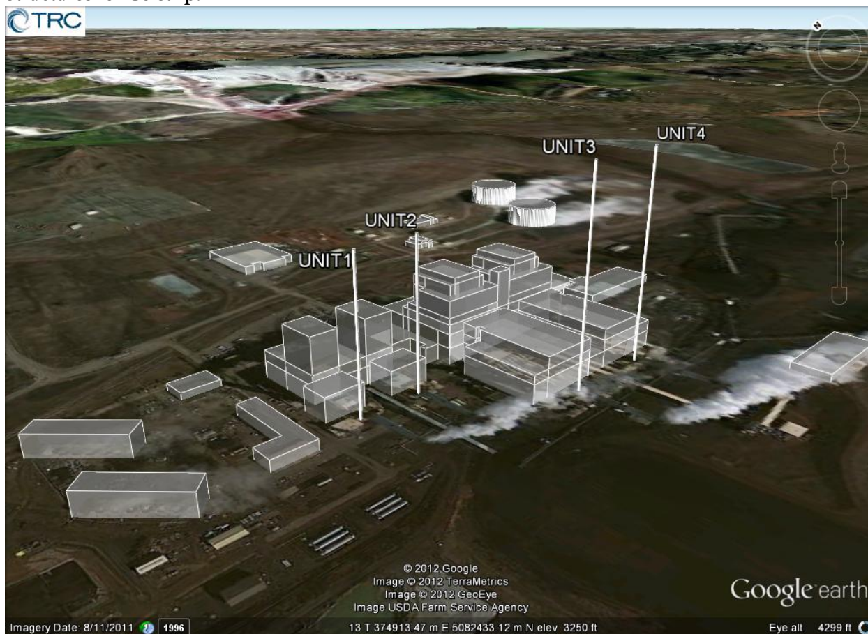
Figure 7. Building Profile Input Program for PRIME (BPIPPRM) Analysis of Stacks and Building Structures for Colstrip.
