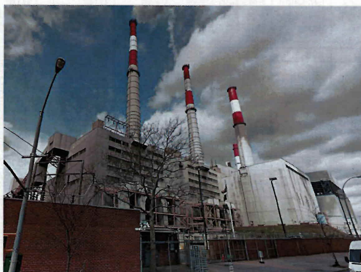
Figure 5-2e: Ravenswood Generating Station
