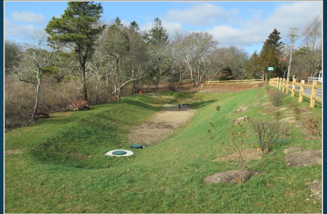
EPA – Chatham BMP Retrofit
