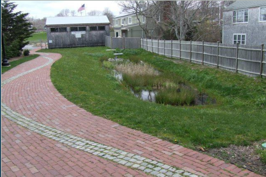
EPA – Hyannis Stormwater BMP
