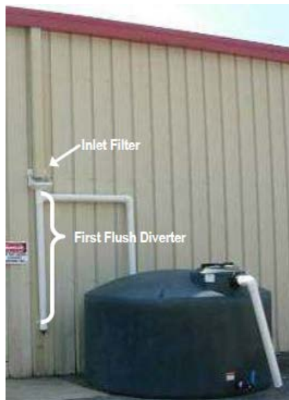
Exhibit 14-10. First Flush Diverter (Credit: NCSU BAE)
