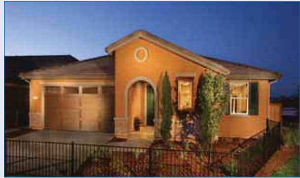
KB Home made history at its Springwood community in Roseville, California last year when it completed construction of the first new homes built to the WaterSense New Homes Specification.
