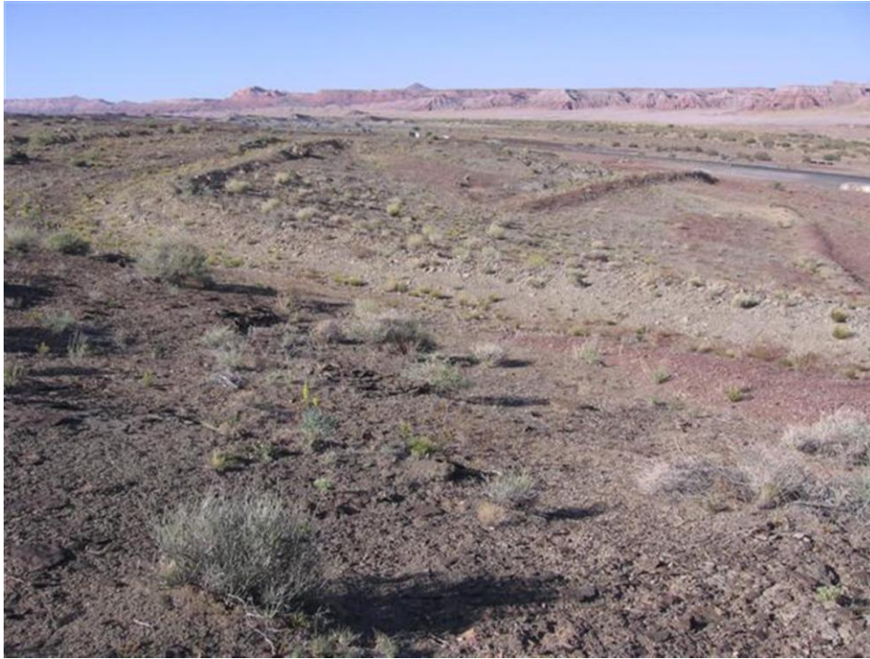
Photo 9: Mine Site #118; Erosion control berms
