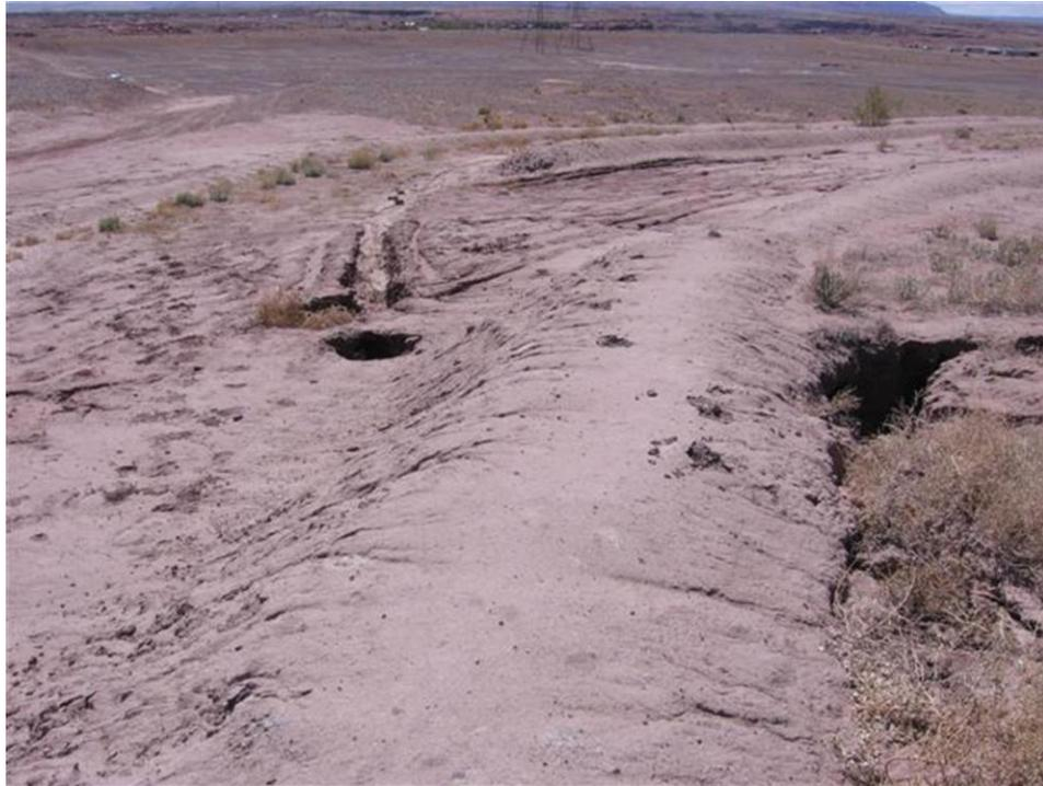
**Photo 2:** Mine Site #124; Compromised erosion control berm
