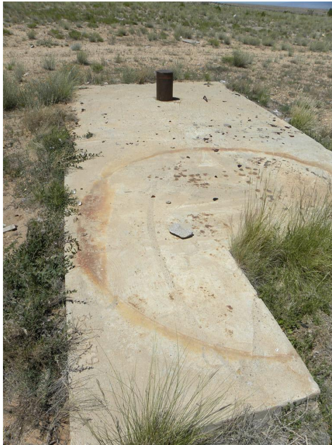
Photo 4. NA-0420 site, concrete pad, labeled 3-29-71
