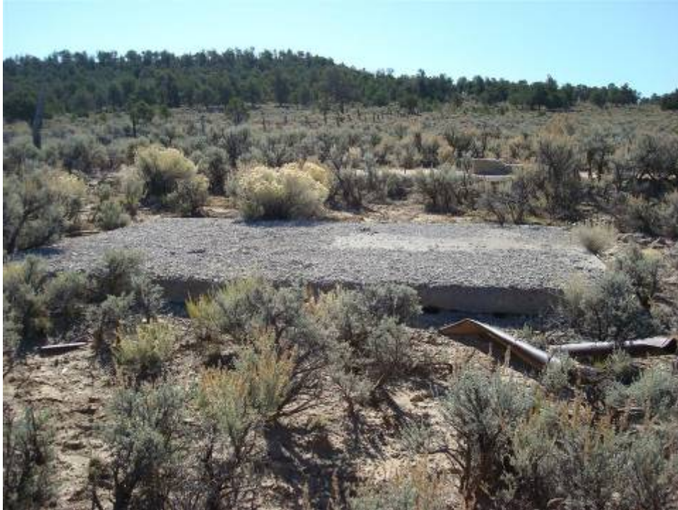
Photo 5. Mac No. 2 Mine site, two concrete pads at the eastern portion of the site
