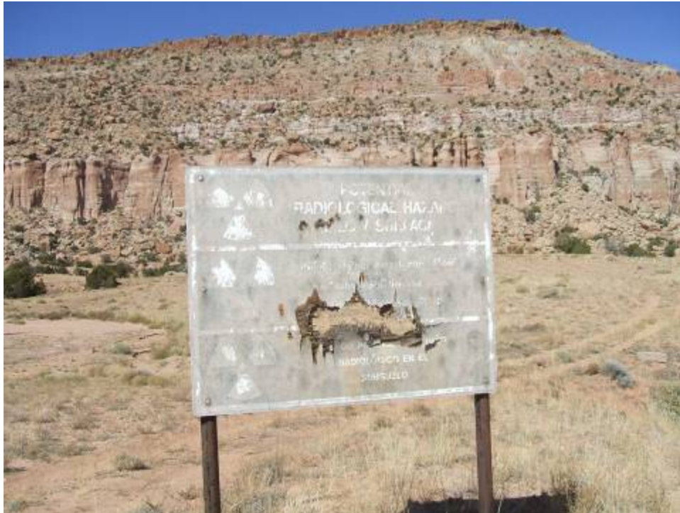
Photo 3. Section 18 mine site “Potential Radiological Hazard” sign, towards the north
