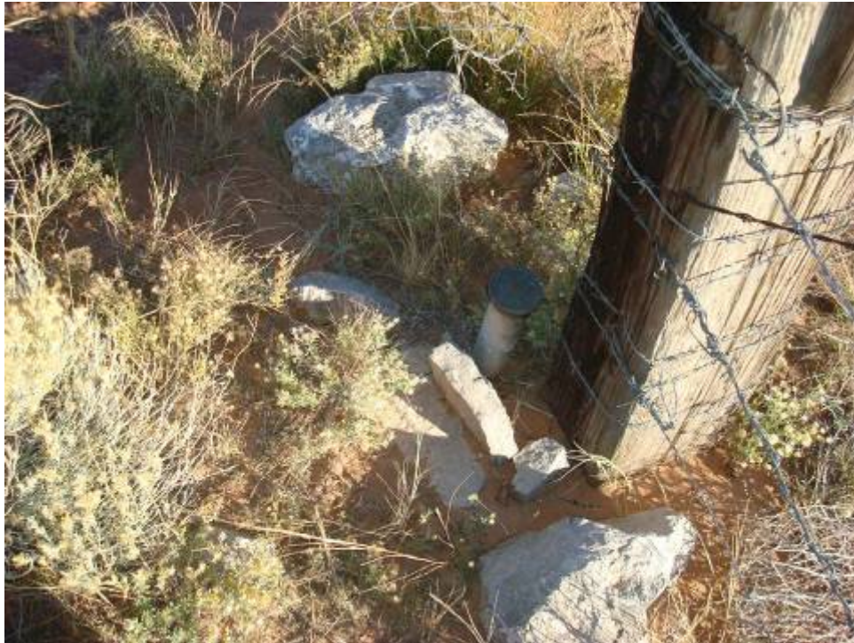
Photo 5. Haystack No 1 Mine site, section corner survey marker
