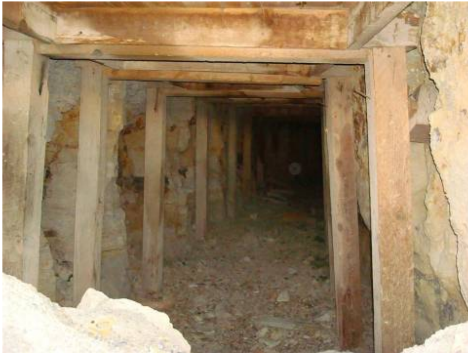
Photo 3. Section 5 Mine site, interior of adit
