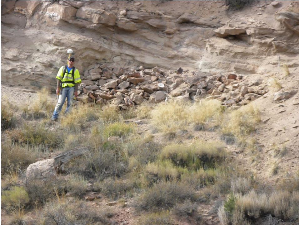
Photo 3. Sealed adit (west)
