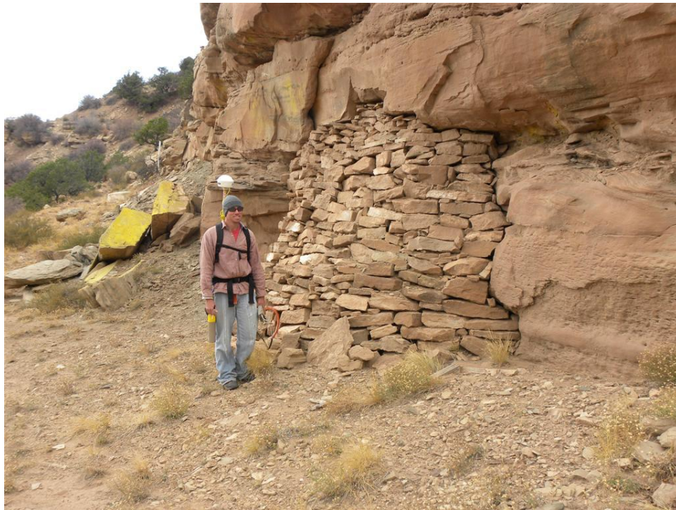
Photo 2. Sealed adit and yellow painted rock
