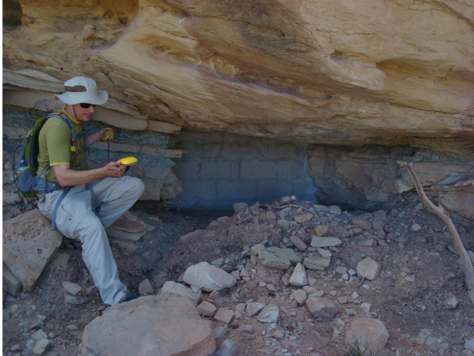
Photo 2. Tsosie 1 mine site, sealed adit
