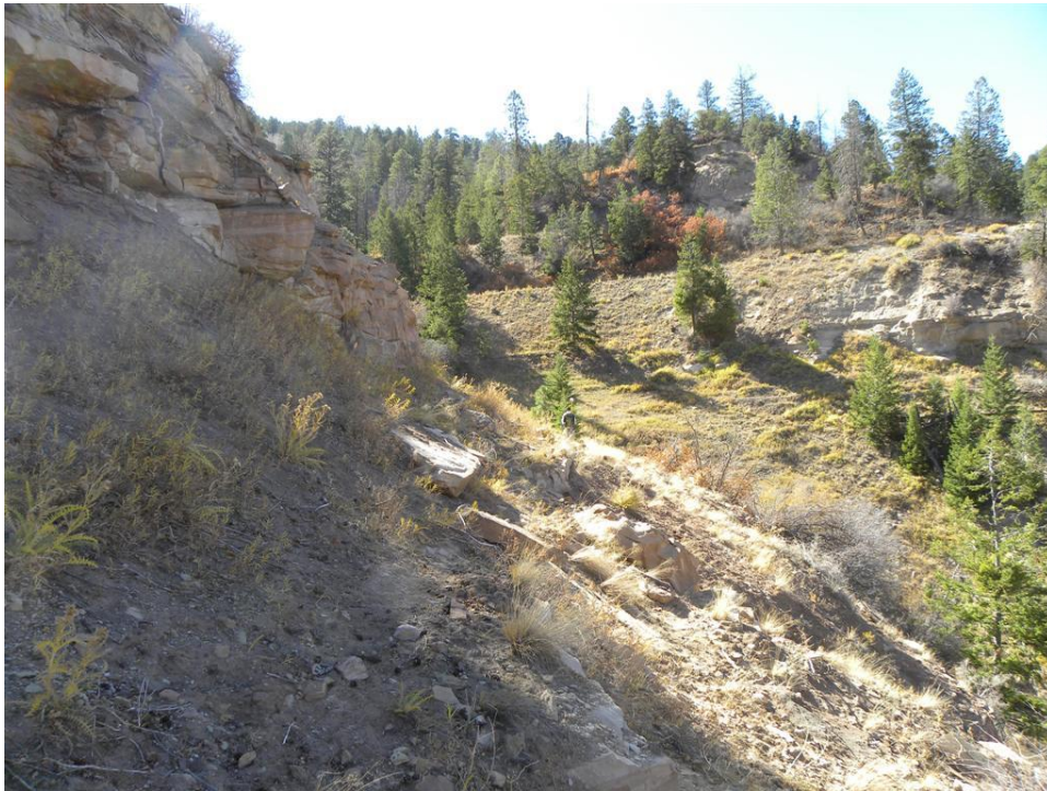
Photo 4. Slope area and waste debris
