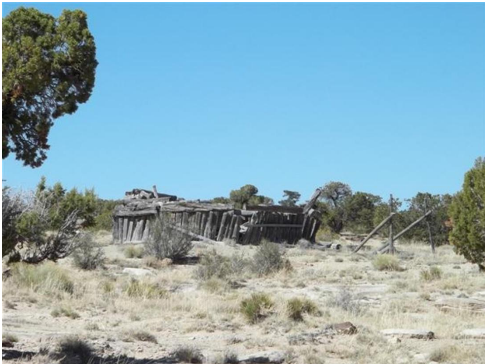
Photo 8: Mine Site #74; Wood structure
