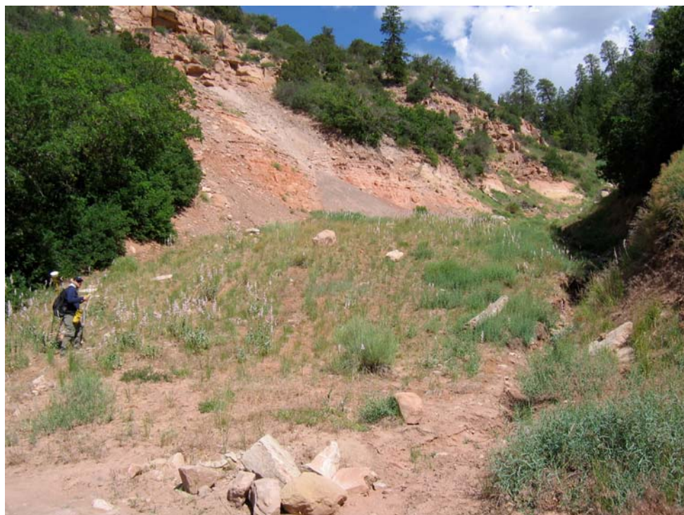
Photo 4: Area reclaimed by the Navajo Abandoned Mines Reclamation Program at Mine 13.
