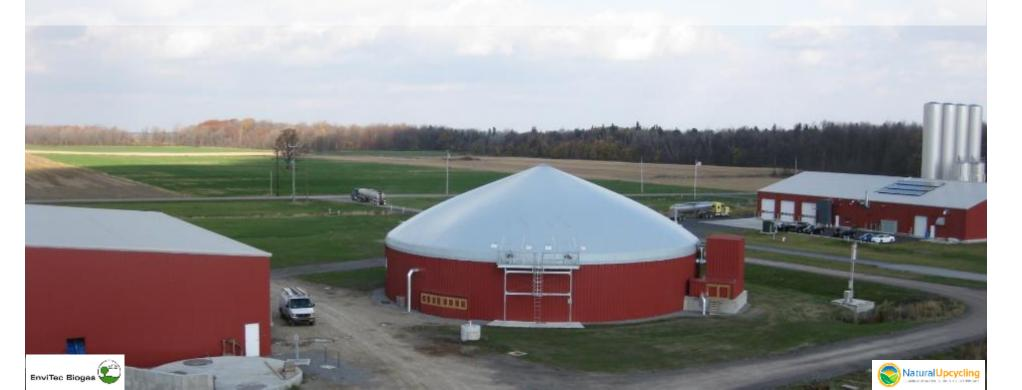
The digester system is designed to receive two different types of substrates; 1)cow manure, and 2) food wastes. It all starts with manure from the Noblehurst dairy cows, which serves as the base volume of material to the tune of approximately 40,000 gallons per day.
