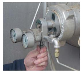
Mizer pilot replacements Reduced leakage ~150 Mcf/yr/valve
