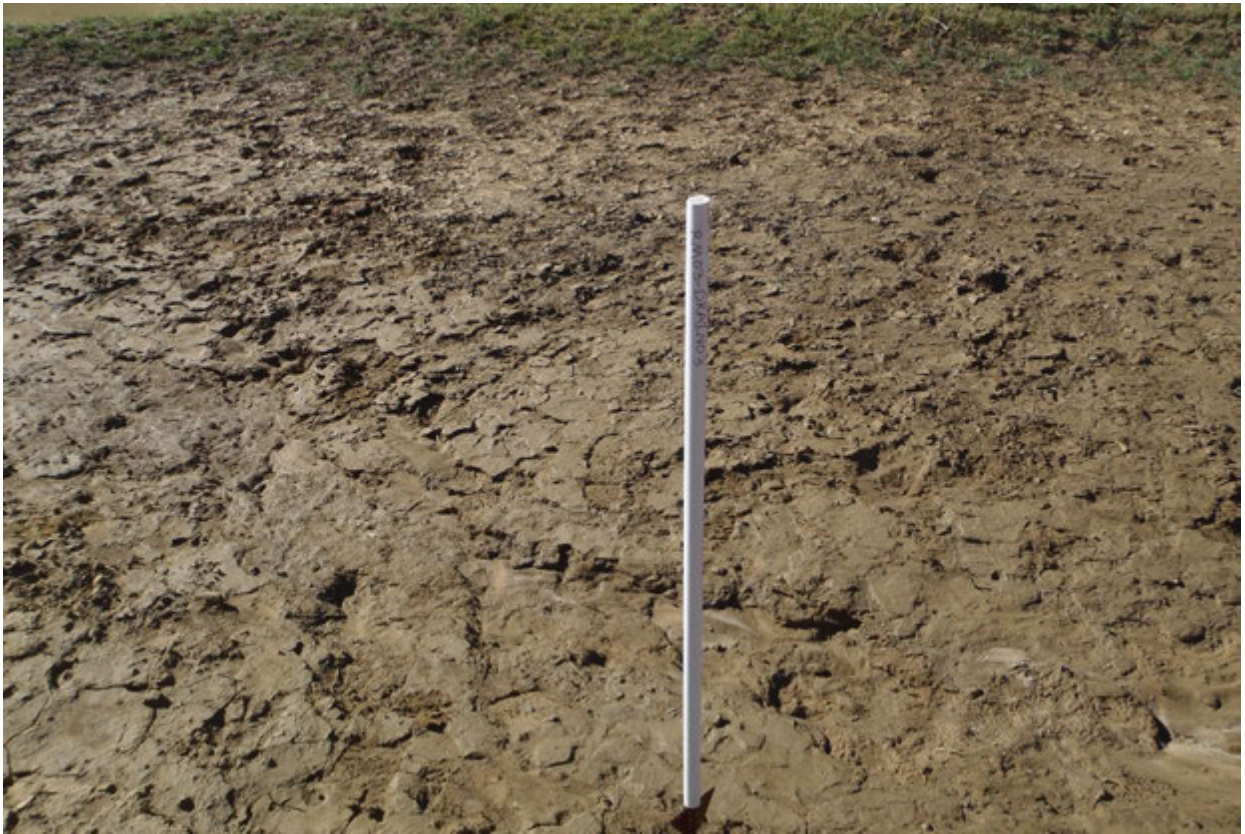
Photo 21: Marking of Soil Borings during Utility Clearance (Boring RM03-DRAIN03 Facing South)
