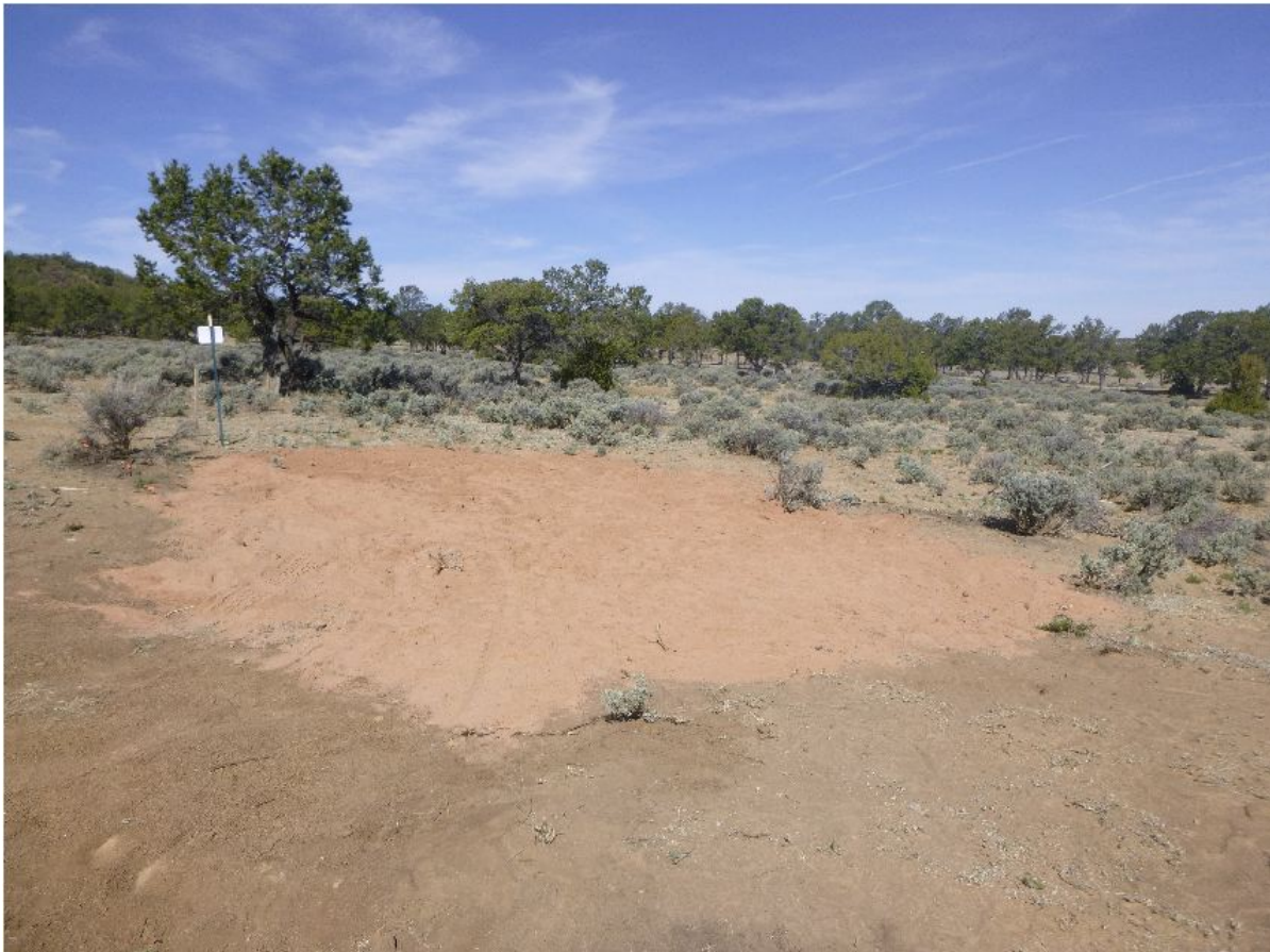
Photo 11: RUBY-018 Vent Closed (Facing West)
