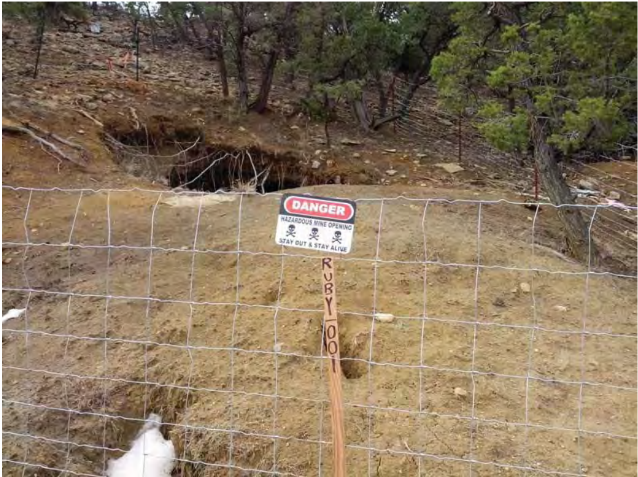
PHOTO 4: Ruby Mine #1 Adit warning signage and fencing. Facing south.
