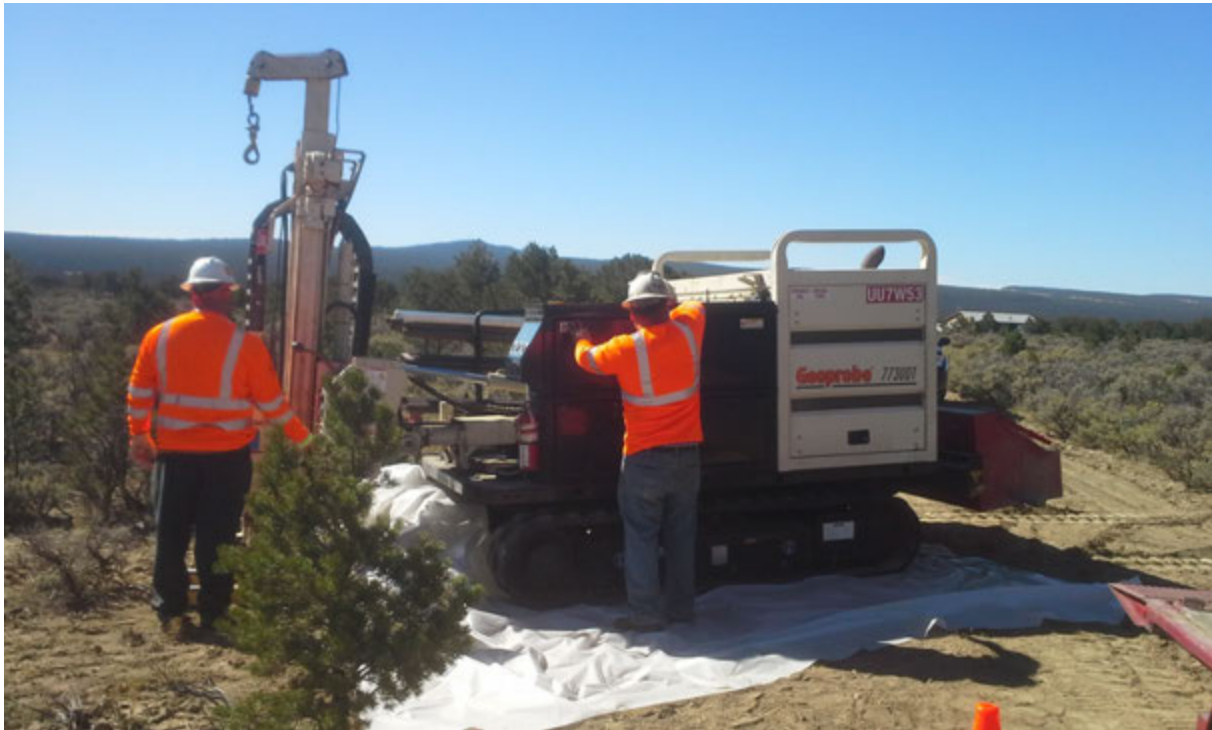
Photo 23: Direct Push Drill Rig Staging (Facing Northwest)
