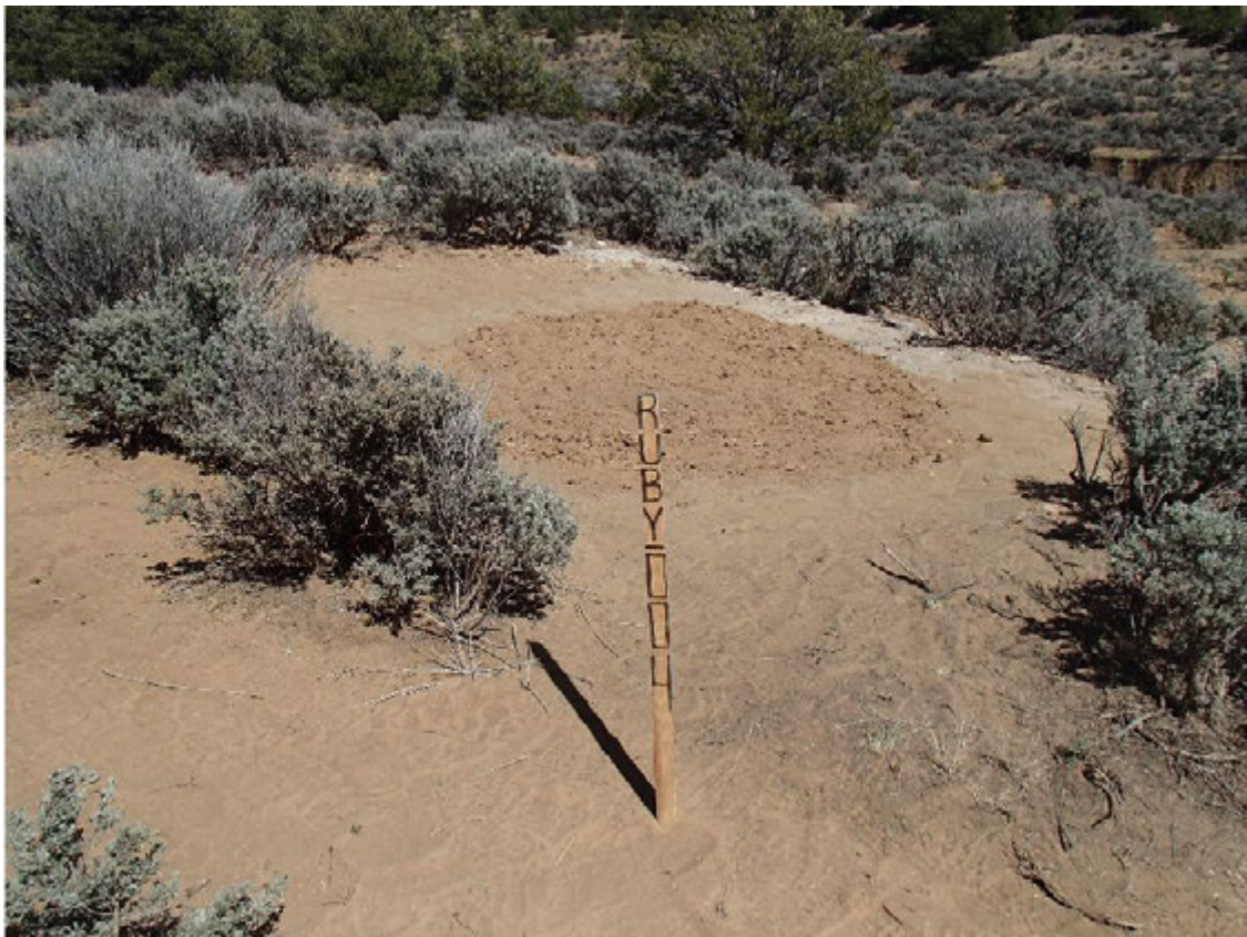
Photo 8: RUBY-004 Vent Closed (Facing Northeast)
