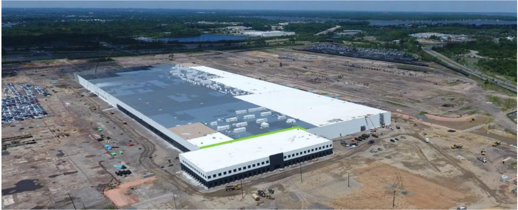
Warehouse Under Construction Photo Credit FCL Builders
