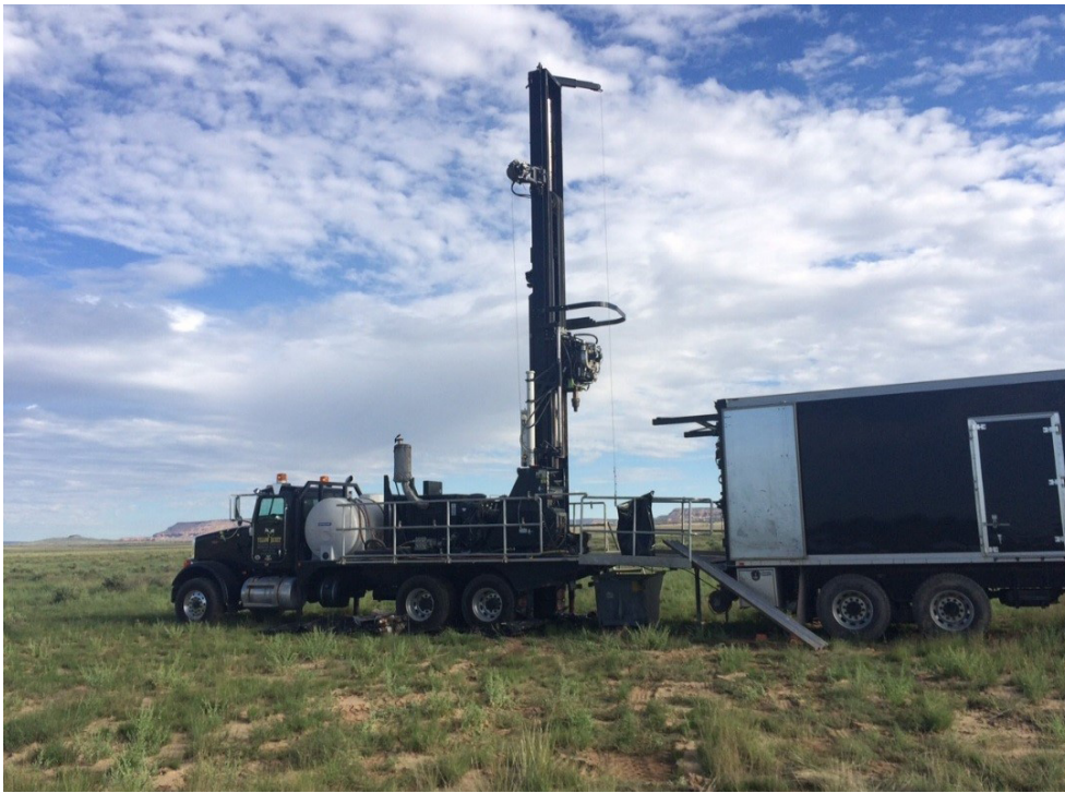
USEPA Conducting Soil and Groundwater Sampling Activities
