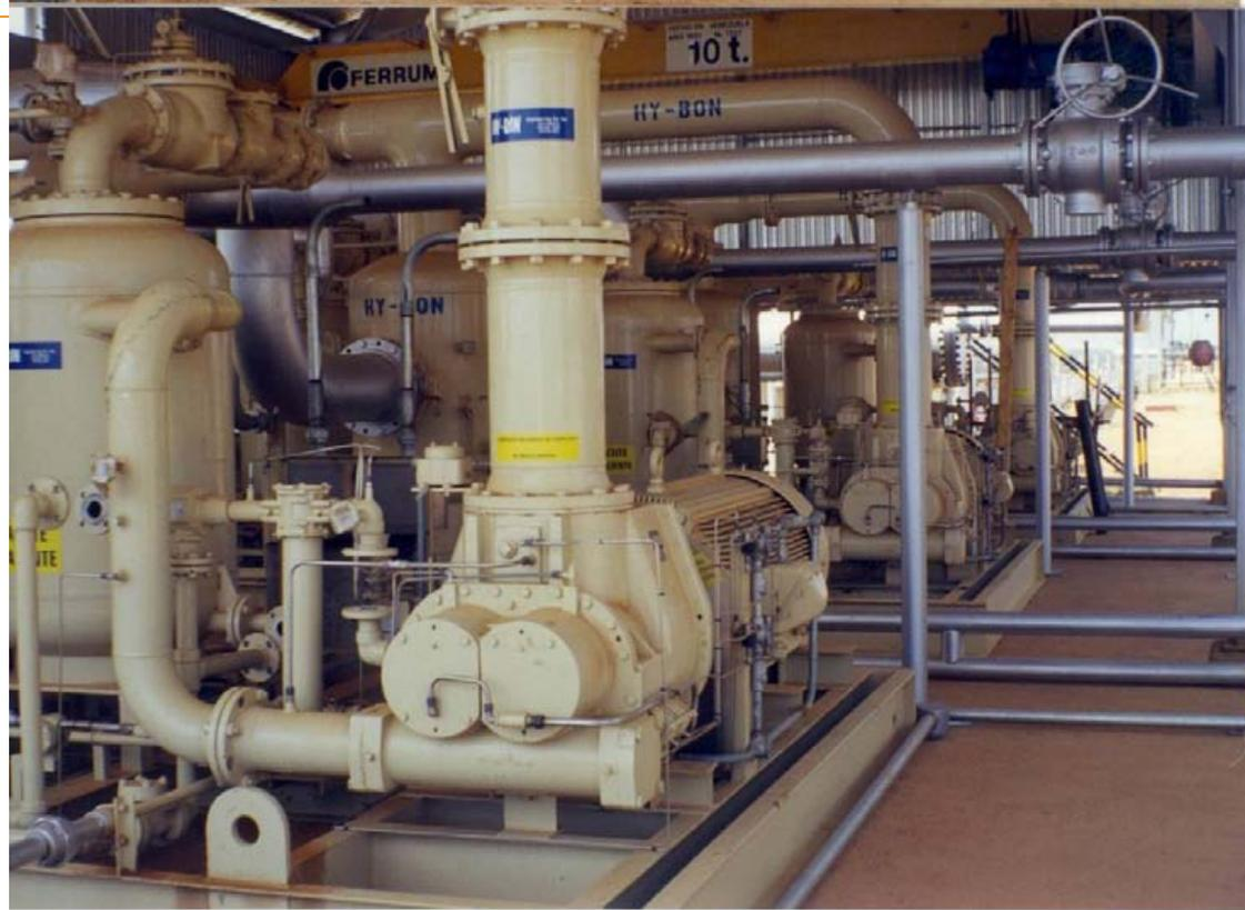
*At this location, three vru compressor packages were set in tandem to move 0,42 MMm<sup>3</sup>D of 630-655 kCal tank vapors.*
