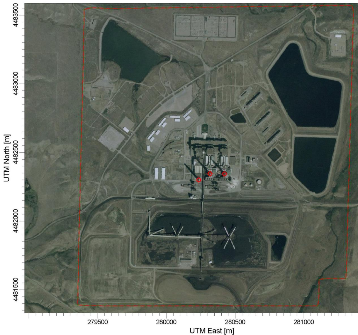
Figure 4. Craig Station Facility Fenceline and Units.
