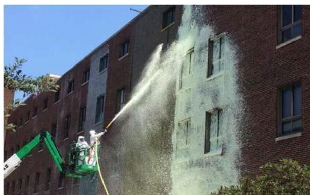
Demonstration of wash down methods for radiologically contaminated buildings Columbus, Ohio 2015
